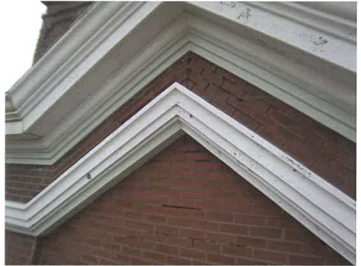
White sheet metal, church front, to patch & repaint
